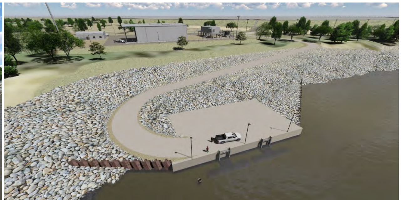
Aerial view of Brazos River Intake
